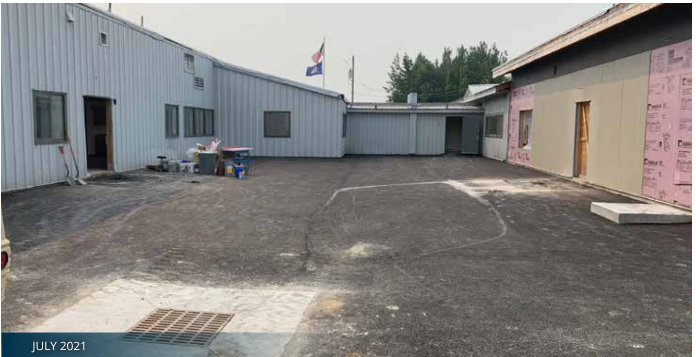
Ready for paving
